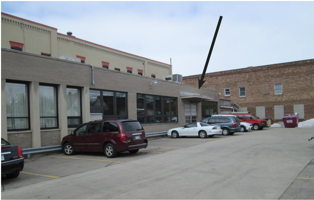
Current view looking northwest from Exchange St at the property line between The Argus-Press and RE/MAX.
