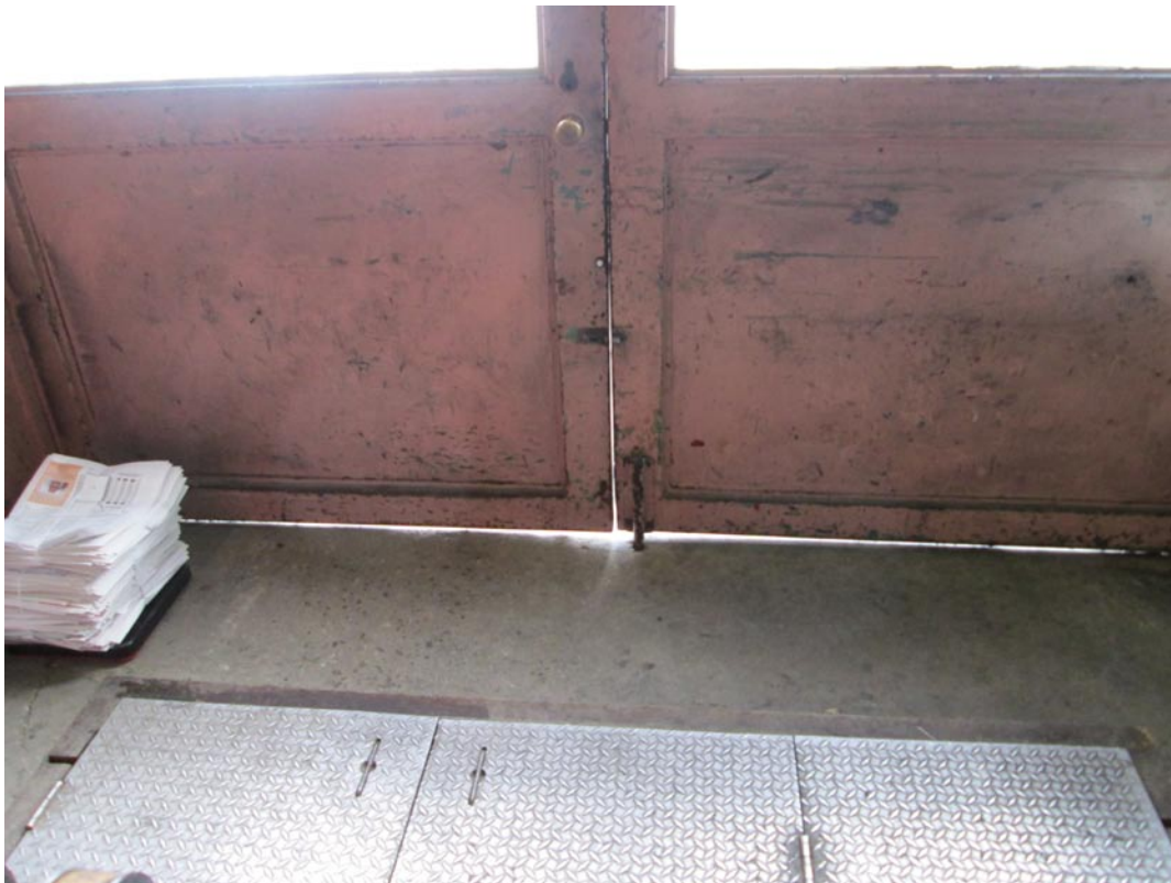
Interior view looking east. This shows the substantial gap at the bottom of the existing doors and also a minor gap between the doors. Both have resulted in terrible heat loss during the winter and a/c loss in the summer.
