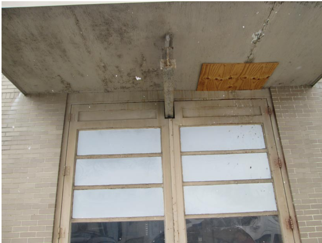
Up angle view looking west from The Argus-Press parking lot. Our door replacement plan includes removing the I-beam that extends outward from the doors and refurbishing the overhanging roof.
